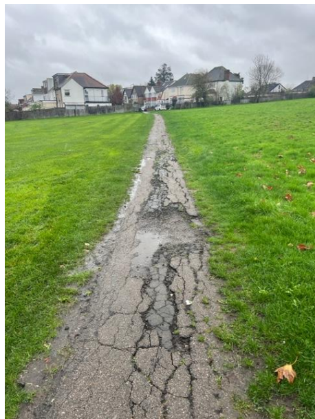
Walking path is not DDA compliant (1.5m wide is the standard required)
