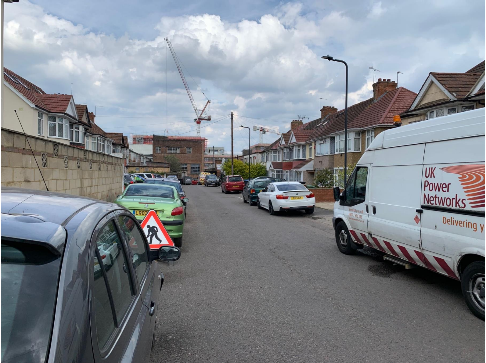
Photo 13: View of south western entrance to site from Woodside End
