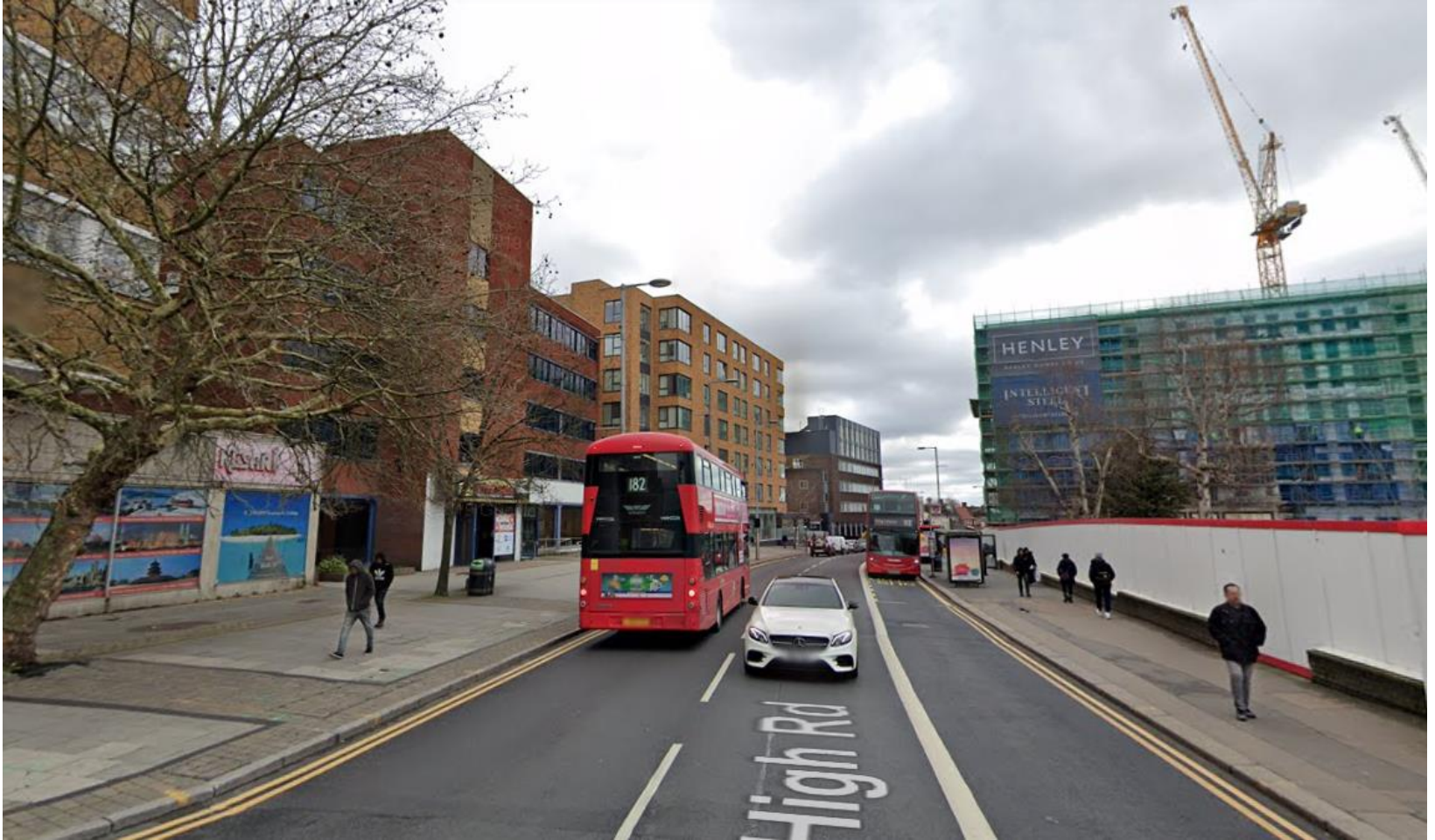
Photo 4: view of site from west
