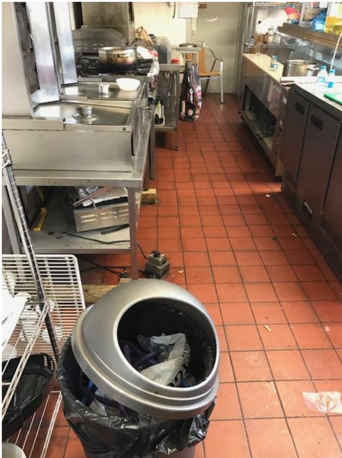
Ground Floor Kitchen – Unhygienic and unsafe kitchen Photo taken on Thursday 13 June 2019 at 12:49hrs
