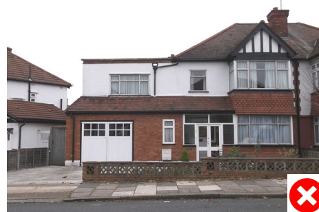
Protruding ground floor and first floor not set back from the main wall
