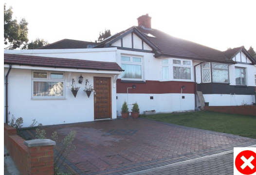
Too wide, protruding, uncharacteristic extension
