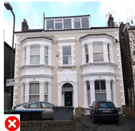
Too large, uncharacteristic front dormer
