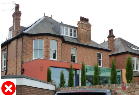
Rear extensions in uncharacteristic materials
