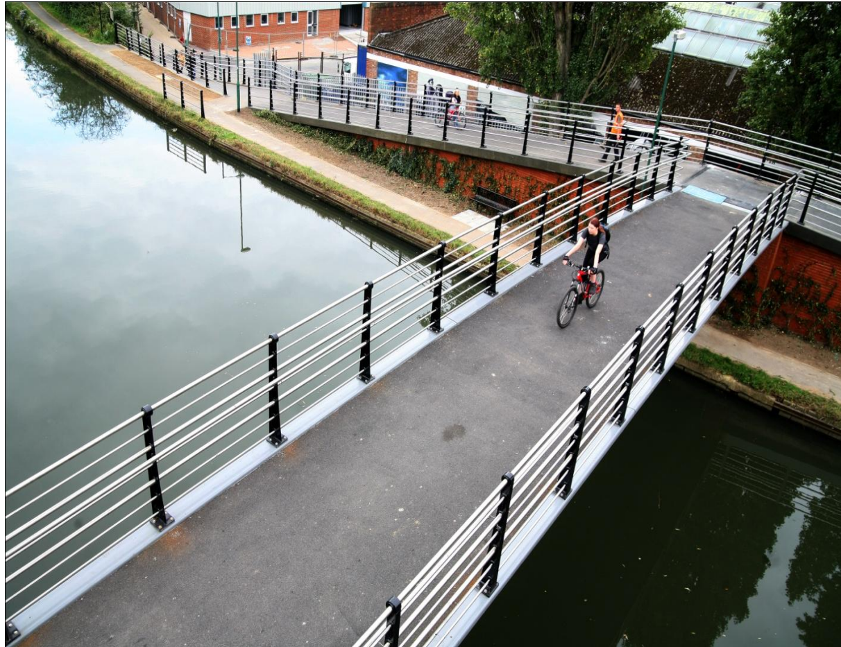
Not only did the new “Grand Union Bridge” facilitate significant improvements for pedestrian and cyclist access to the Grand Union Canal, near Alpertons, it was unique in its overarching objectives and aspirations to design out crime.
