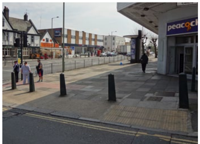
Cluttered pedestrian footways
