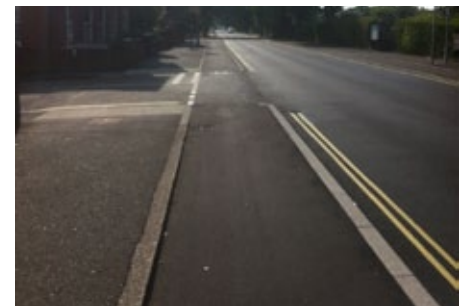
Old Shoreham Road in Brighton, where high quality segregated cycleways have been provided;
