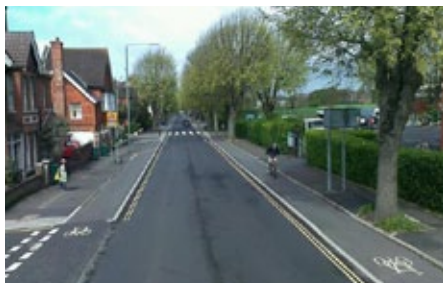
1. Cycle Facilities - Old Shoreham Road
