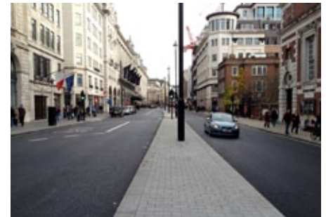
Piccadilly, where two-way traffic has been reintroduced, guardrails have been removed and a median strip provided;
