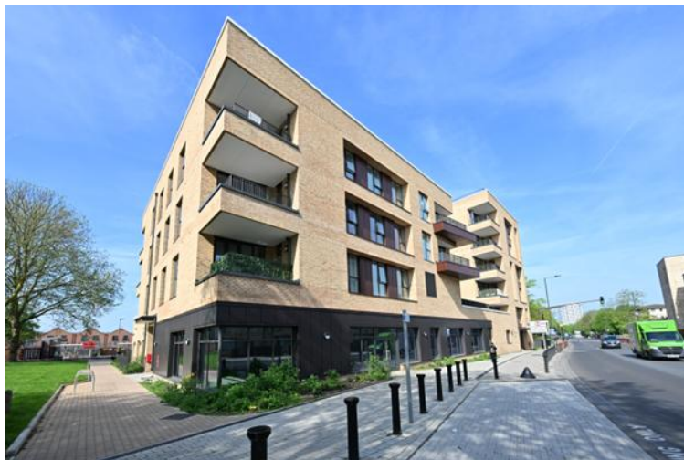
Photograph of Roy Smith House, Stonebridge (Source: LBB)
