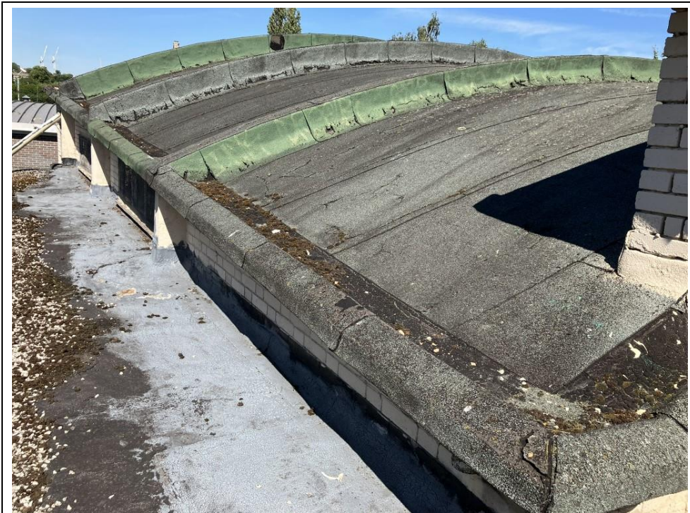
4. Central section, mineral felt barrel roof.
