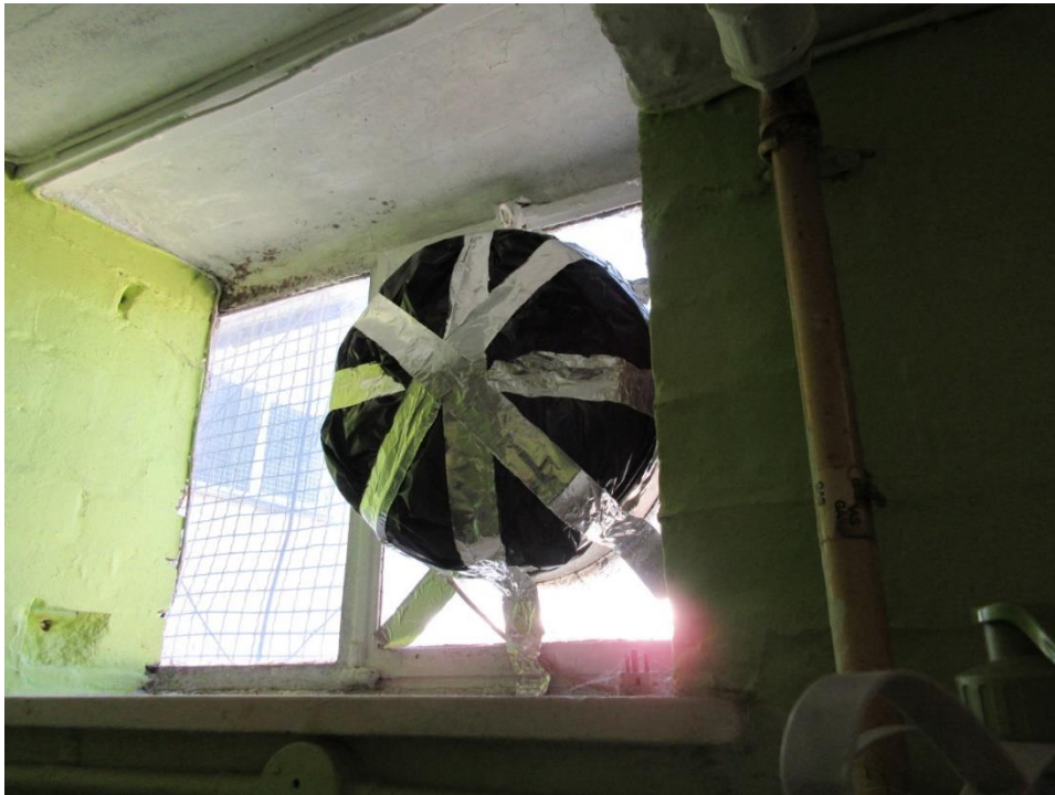
63. Kitchen extract fan is isolated and temporarily covered
