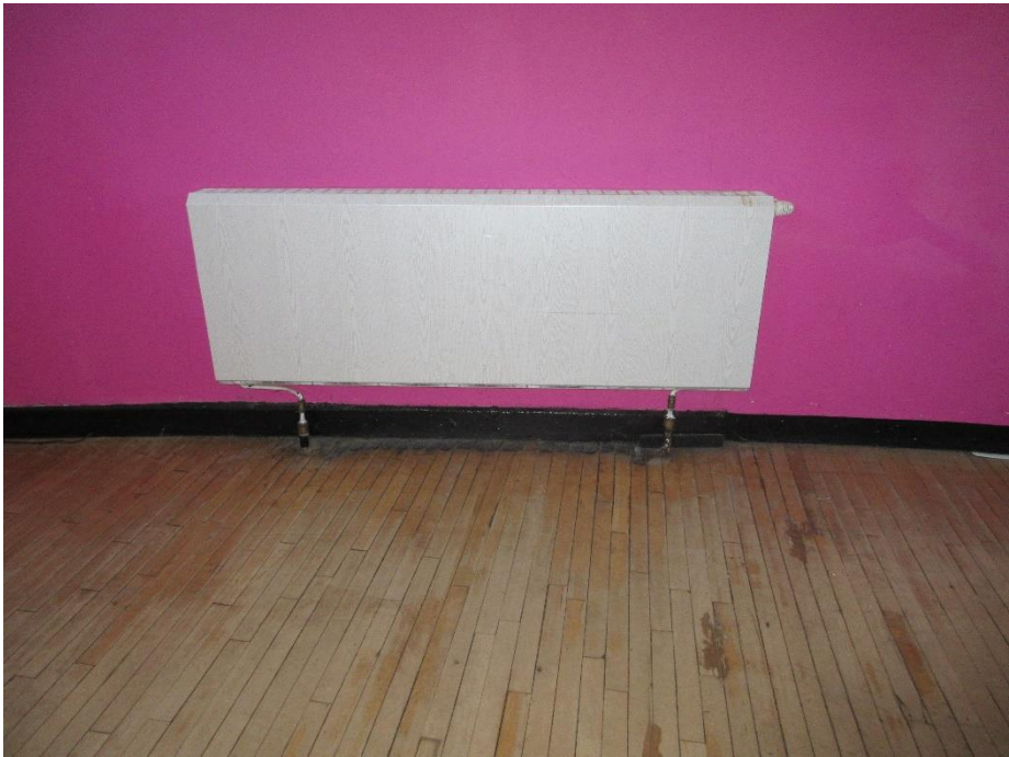
55. Typical radiator in the main hall, provided with LST cover
