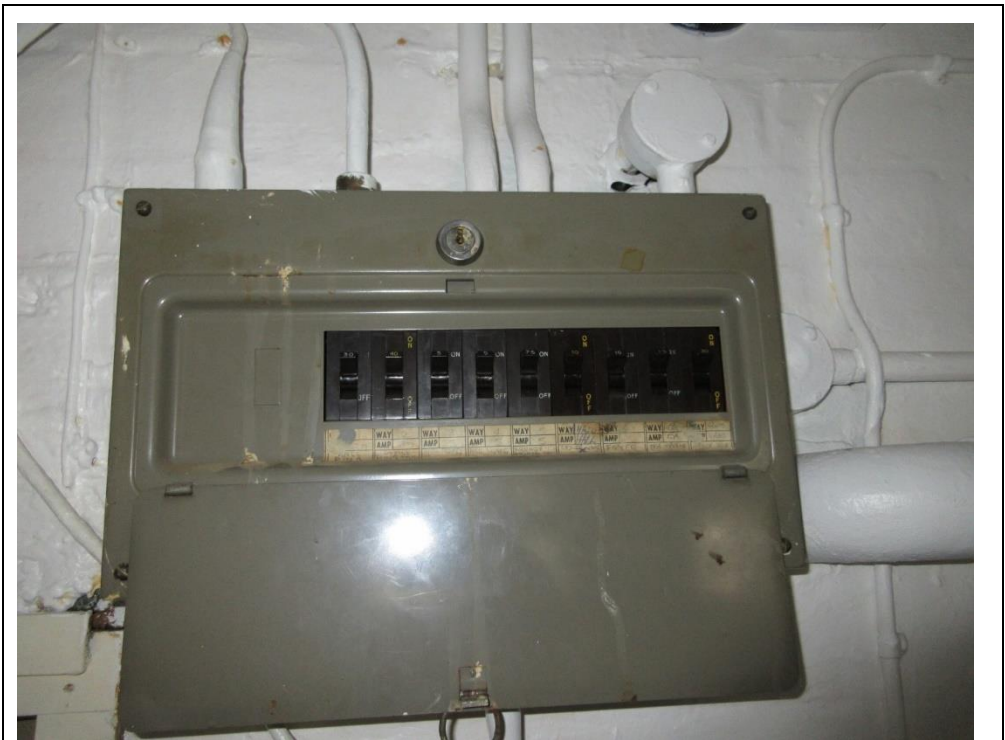
65. Typical aged distribution board, no circuit schedule
