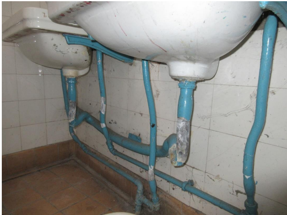
62. Lead pipework on the domestic and waste services. Waste pipe is unsupported and now not laid to a fall
