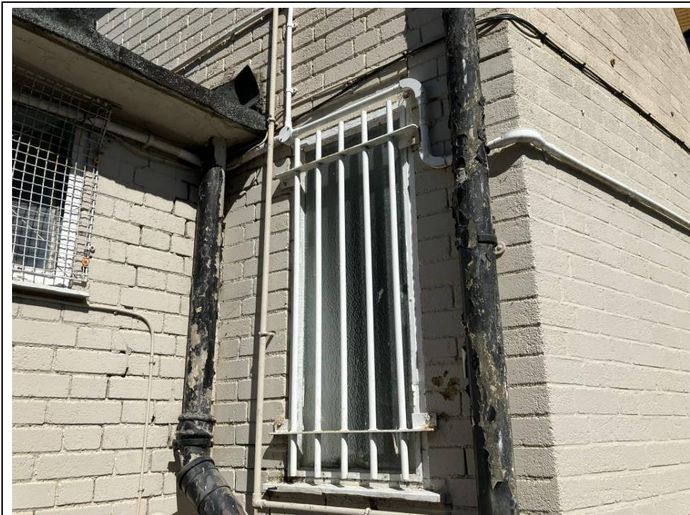
15. Front elevation central section, cast iron downpipes and window bars.
