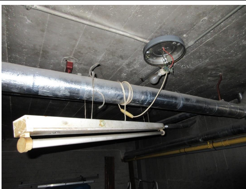
67. Typical poor lighting modification / repair on site
