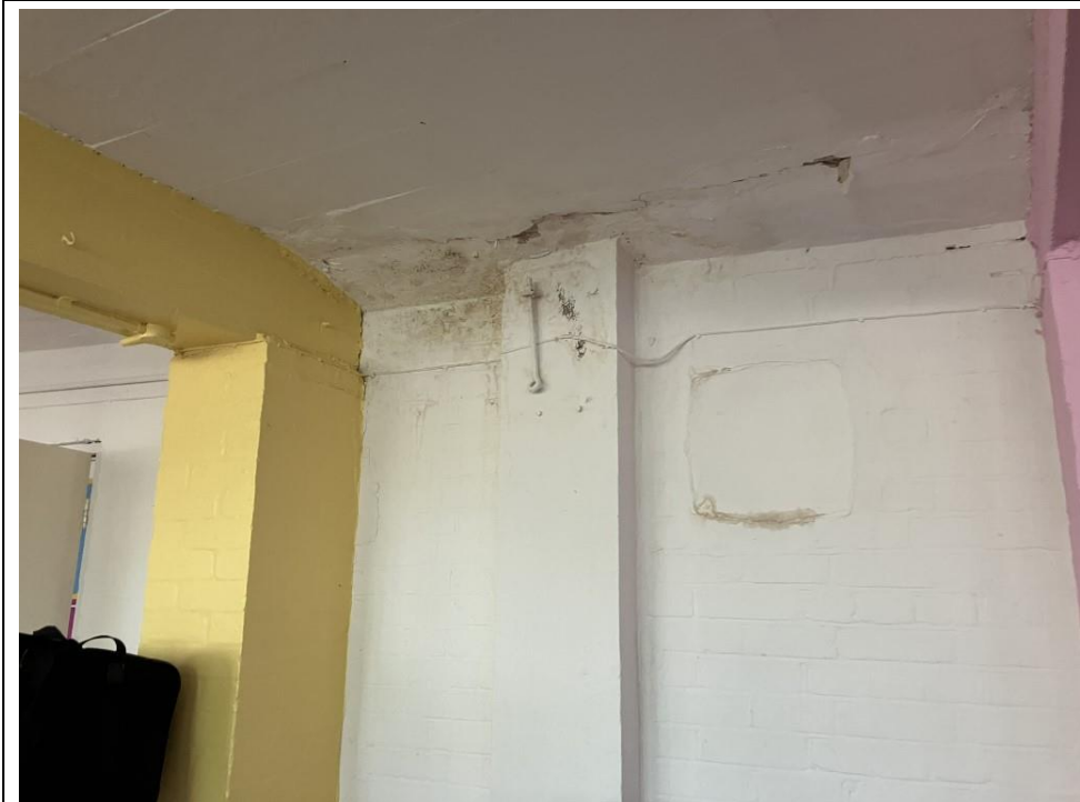
26. Ground floor east section, typical water ingress stain.
