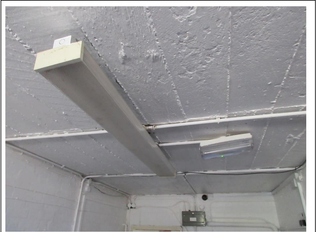
66. Typical aged fluorescent lighting and emergency lighting
