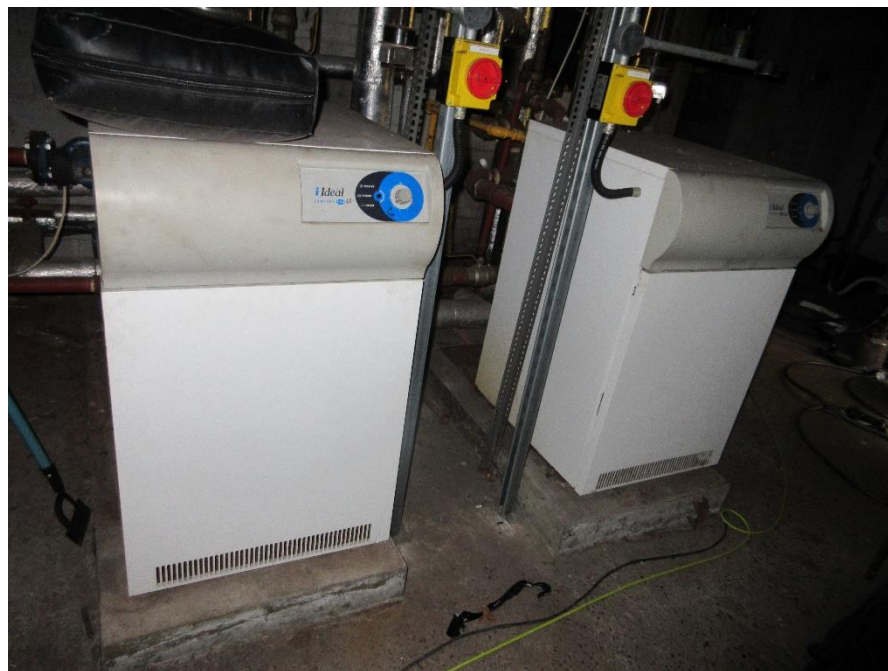
50. Gas fired boilers in the basement plant room, isolated and not operational at the time of our survey.
