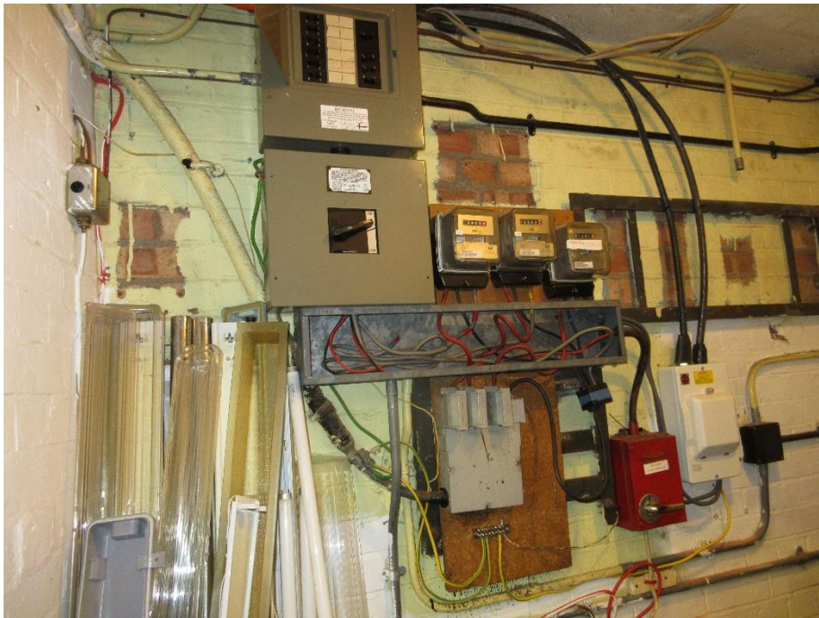
64. Incoming electrical supply, utility meter and distribution board
