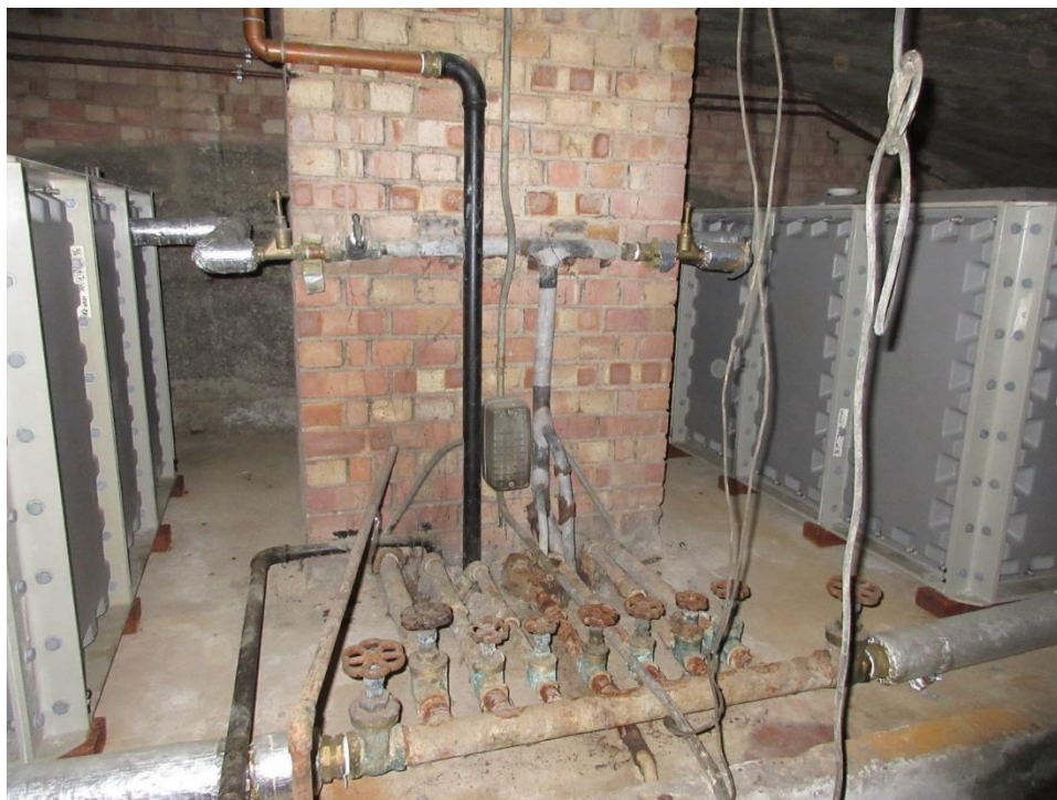
61. Mixture of pipework materials, lead, copper, steel
