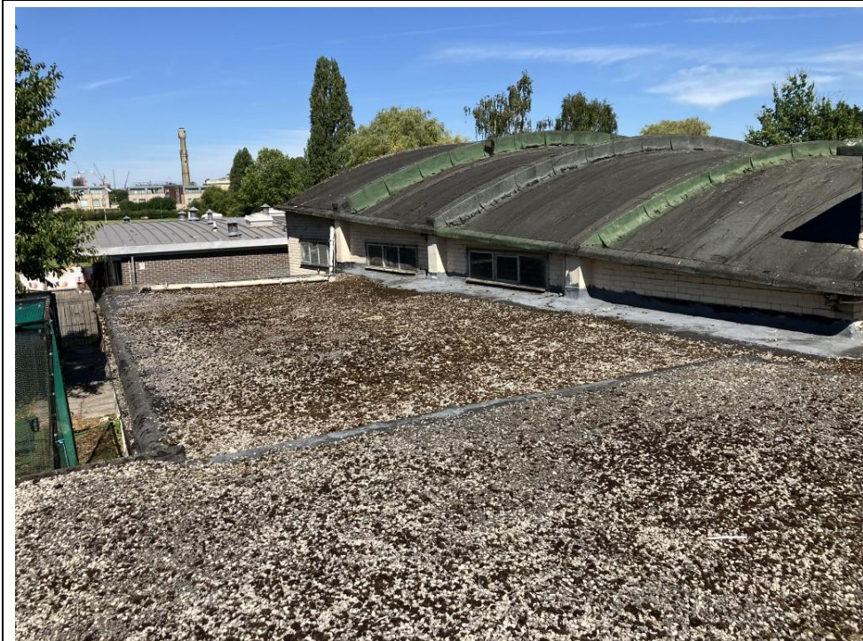
3. East section, mineral felt flat roof.
