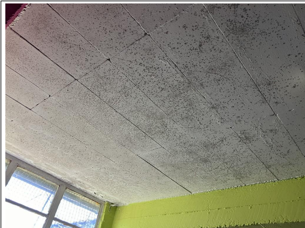
25. Ground floor east section, typical mould growth.
