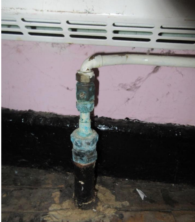
56. LTHW connections on the LST radiators are exposed and some are show signs of leaks / corrosion
