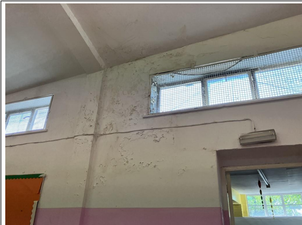
31. Ground floor central section, stained and flaking paint finish.
