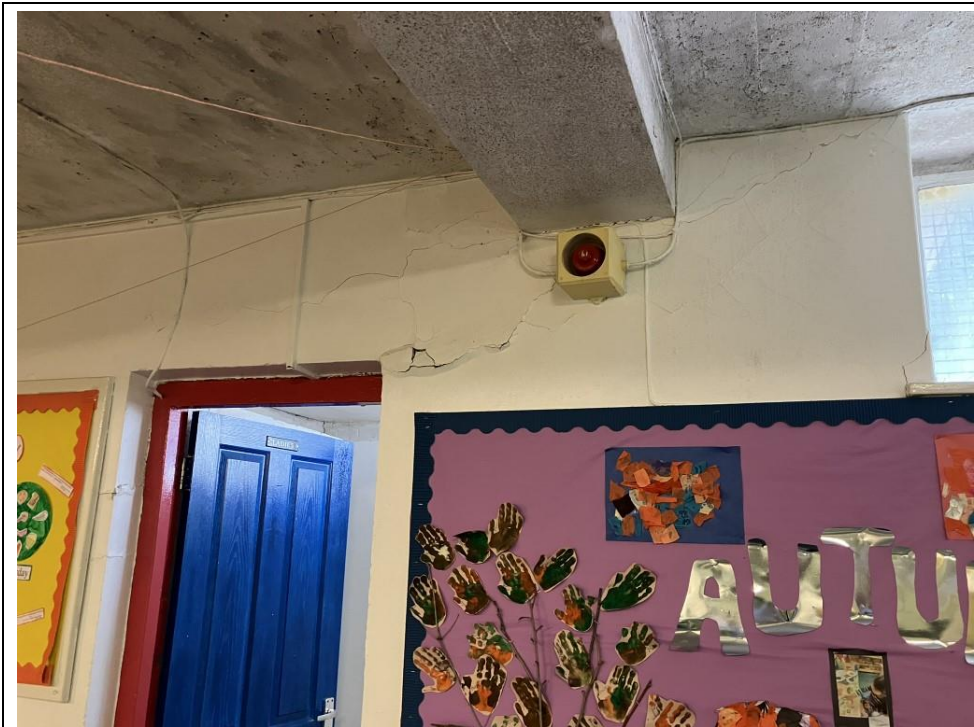
37. Ground floor west section, indicative cracking.
