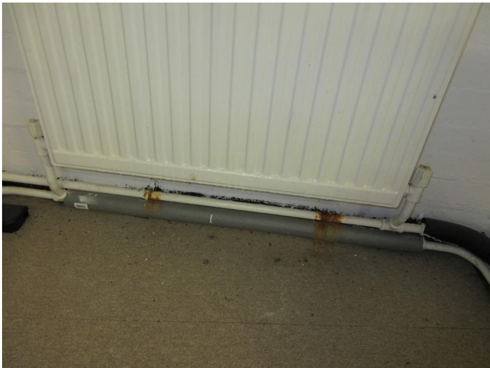
57. Other signs of leaks / corrosion on the LTHW system
