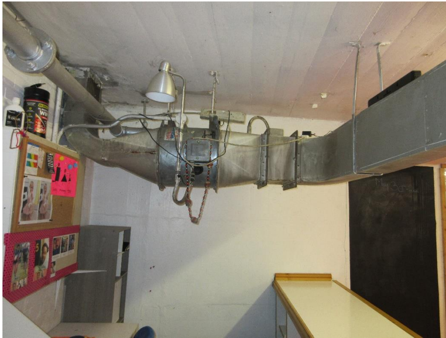
53. Extract fan serving the basement
