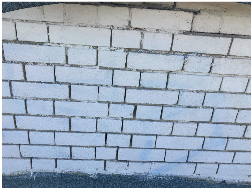
9. Central section (roof level), indicative failed pointing.
