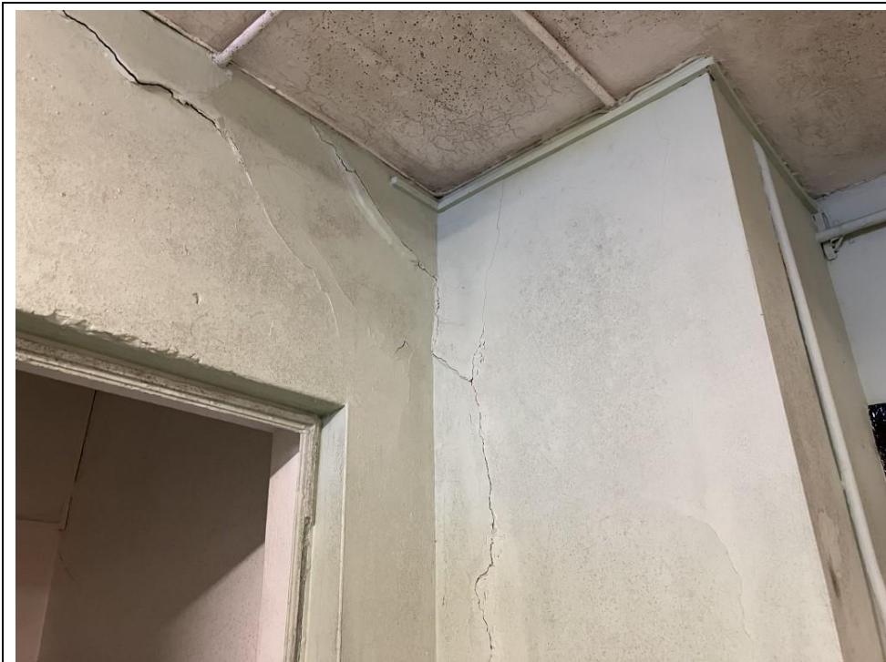
35. Ground floor west section, indicative mould growth and cracking.
