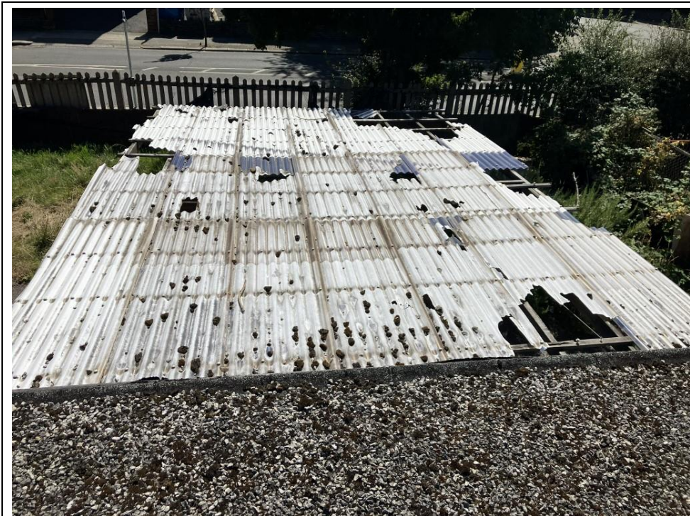
2. Projecting canopy PVC roof to front elevation east section.
