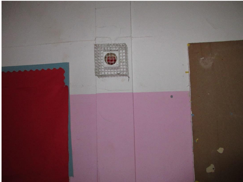
70. Fire alarm sounder/beacon
