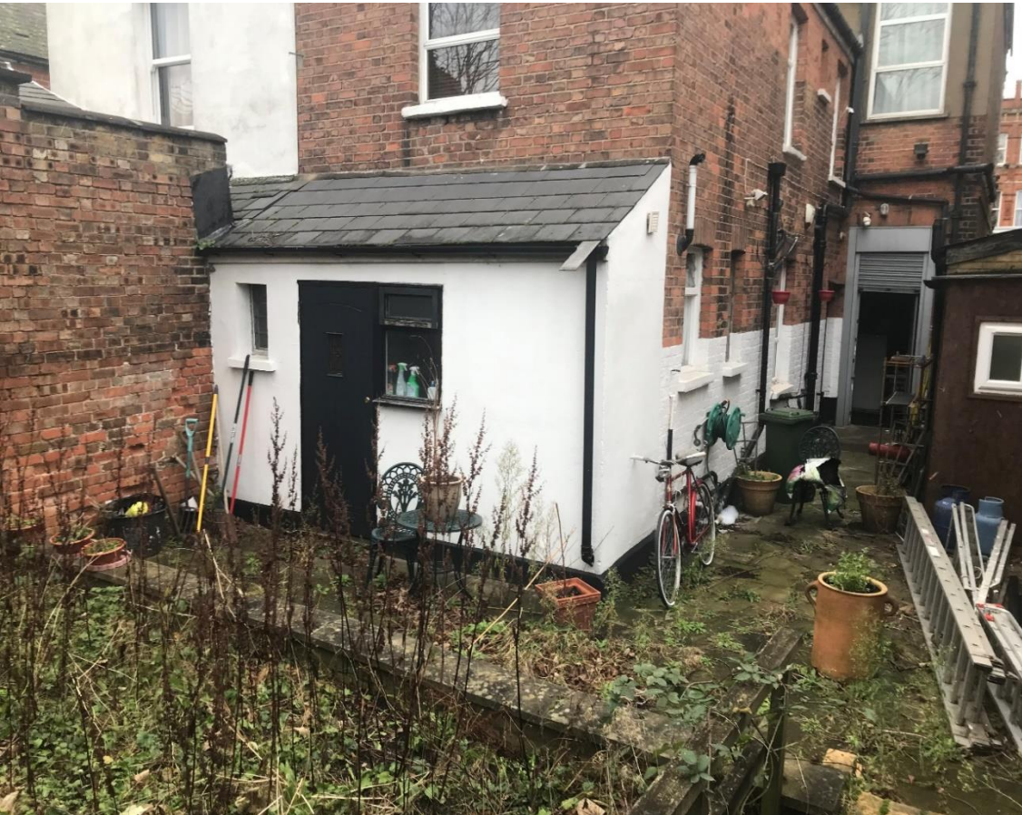
Rear of Premises/ Toilet Area.
