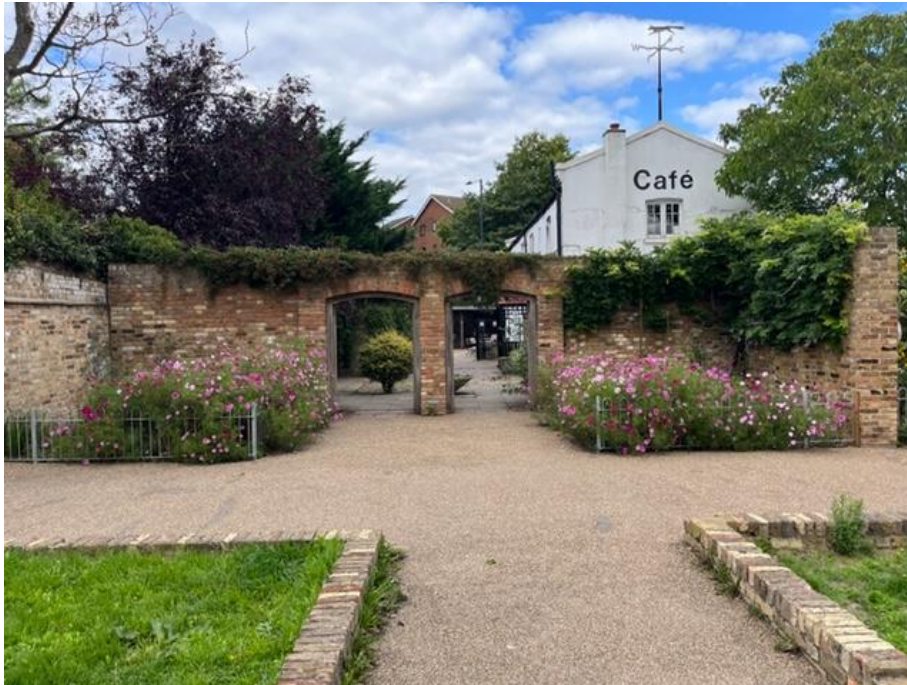
Completed Gladstone Park S106 Works (Source: LBB)
