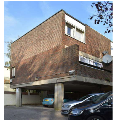
3. EXISTING MAISONETTE BLOCK WHICH RESTRICTS ACCESS FROM EXETER ROAD
