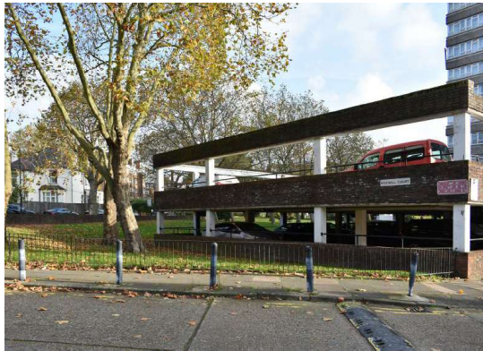
7. TWO STOREY OPEN SIDED CAR PARK LOCATED WITHIN AREA MOST SUITABLE FOR REDEVELOPMENT. EXTENT OF PARKING PROVISION TO BE RE-PROVIDED WILL DICTATE PROPOSED BUILDING FOOTPRINT AND QUANTUM OF ACCOMMODATION.
