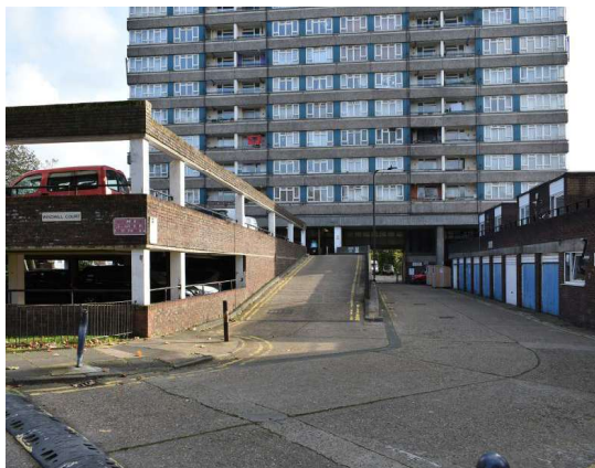
4. CAR PARK RAMP AND GARAGES DOMINATE APPROACH TO WINDMILL COURT. PUBLIC REALM SUFFERS FROM LACK OF PASSIVE SURVEILLANCE AND POOR LEGIBILITY FOR VISITORS.
