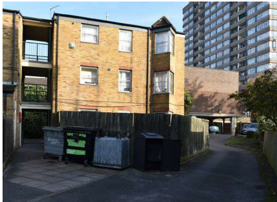
2. VEHICULAR ACCESS FROM EXETER ROAD IS NOT CURRENTLY SUITABLE FOR REFUSE VEHICLES, FIRE APPLIANCES OR CONSTRUCTION ACCESS. WHICH PRECLUDES DEVELOPMENT OF PLOT BEHIND MAISONNETTES.
