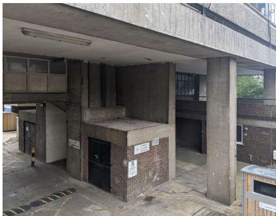
9. POOR QUALITY PUBLIC REALM AND VISUALLY DOMINANT BIN STORES RESULT IN AN UNINVITING ENTRANCE TO THE EXISTING TOWER
