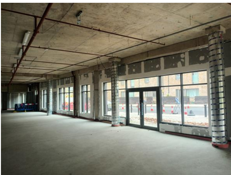
Photograph of Roy Smith House community space fit out (Source: LBB)
