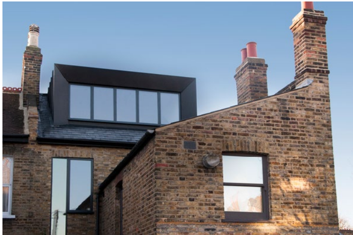
Example: 30 Lampmead Road, N4. Dormer extension sits behind the existing building line, does not follow the outrigger, and uses well-detailed standing seam metal with generous glazing.
