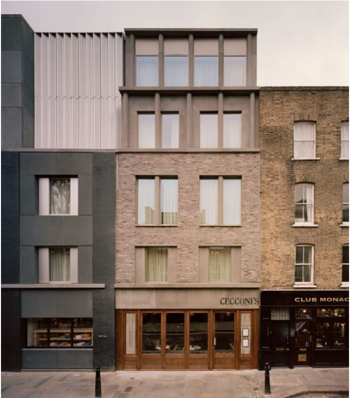
▲ Example: Redchurch Townhouse in Shoreditch by 31 44 Architects. Commercial unit at ground floor is carefully aligned to neighbouring existing buildings, while upper storeys and glazing relate closely to adjacent buildings. Contemporary material treatment is distinct from historic neighbours.
