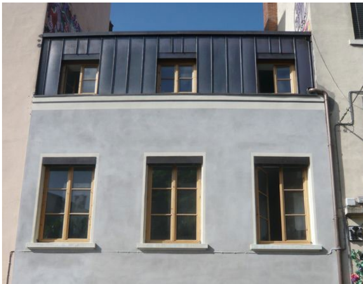
Example: Apartment building in Lyon by Fabien Perret Architectes. Mansard extension sits behind the elevation of the existing building. Recessed windows within a dark standing seam metal recede visually from the lower elevations.
