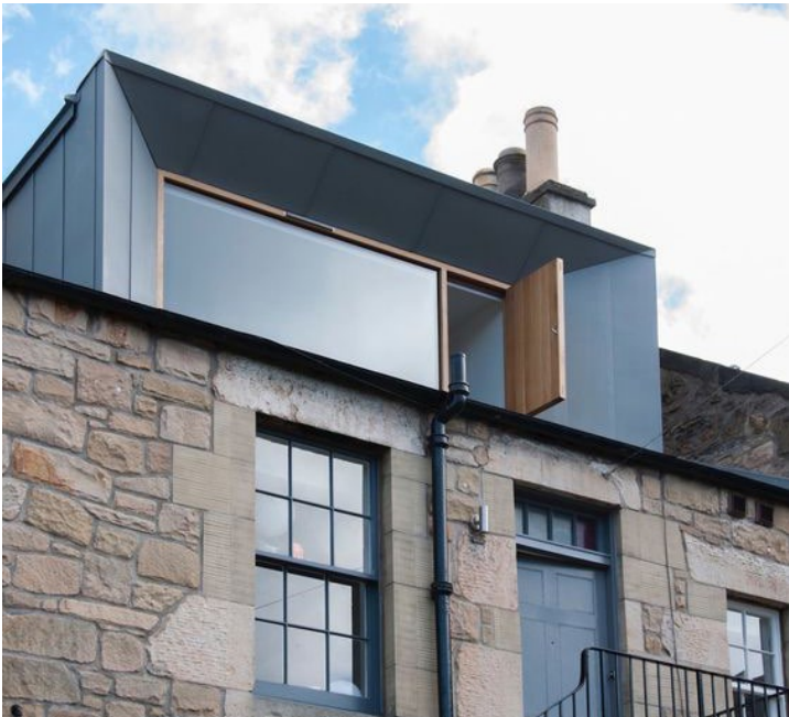
Example: Roof extension in Edinburgh by Konishi Gaffney Architects. Bold, simple volume using standing seam metal establishes a sympathetic contrast with the existing building.
