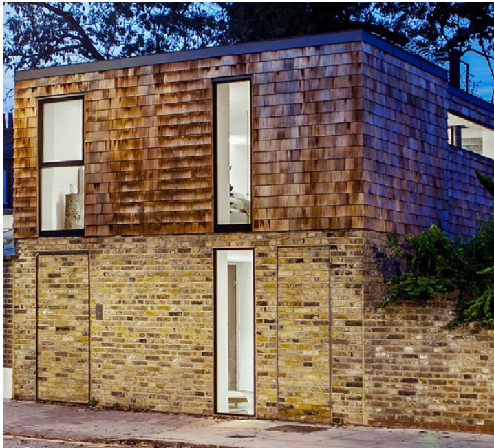
Example: Development in Dalston by Marta Nowicka. Simple, low profile volume in timber shingle contrasts gently with the brick wall below. Openings align between floors for an ordered composition.
