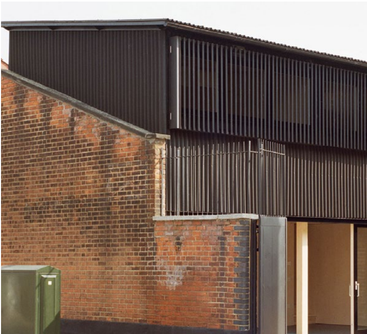
Example: Windsor Road house by Russell Jones Architects. Low profile volume in contemporary vertical timber cladding does not distort proportions of existing wall to street.
