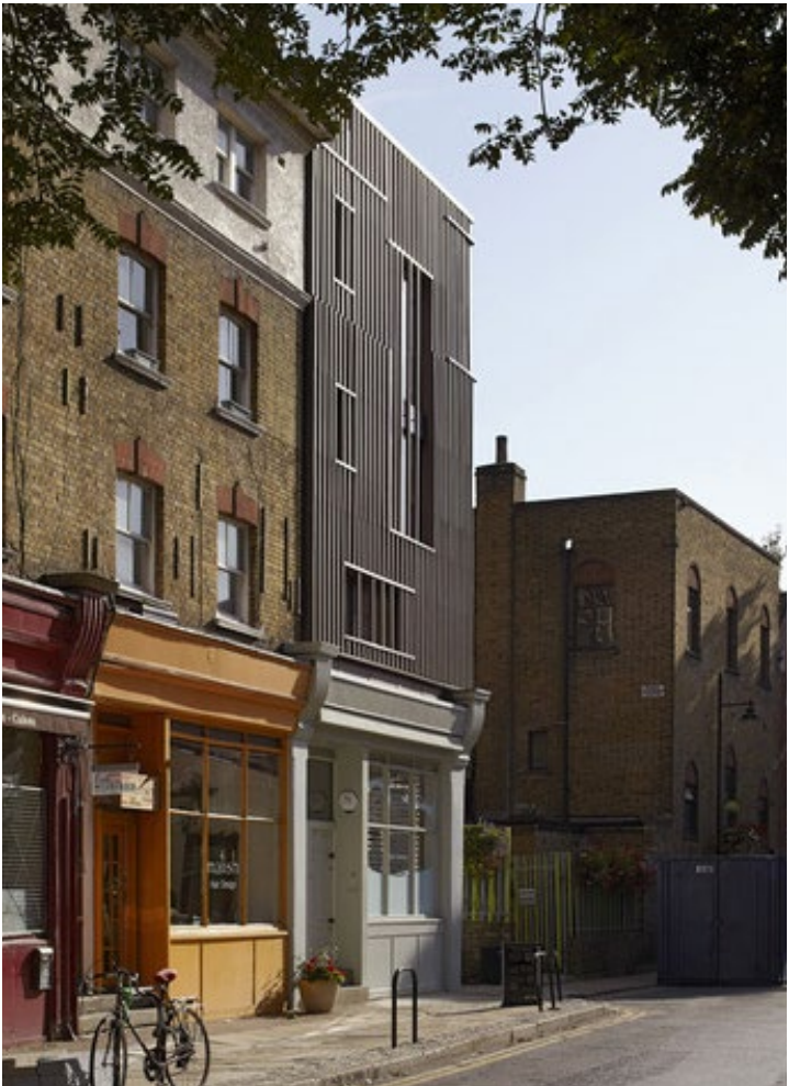
Example: Alex Monroe Studio, Southwark, by DSDHA. Extension to single storey retail unit picks up on eaves and window heights of adjoining terrace, uses contemporary material treatment to achieve clear distinction from host building.
