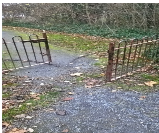
Gates scoring the path surface at Coronation Gardens
