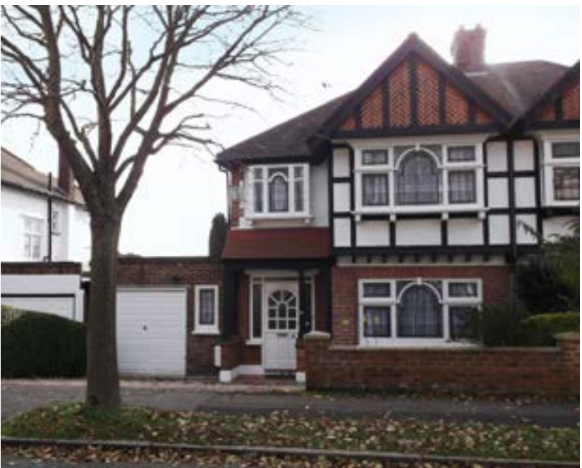
Figure 22: Decorative features at Sudbury Court
