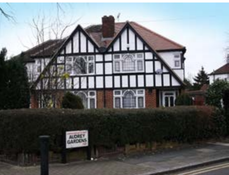
Figure 24: Half timbering at Sudbury Court
