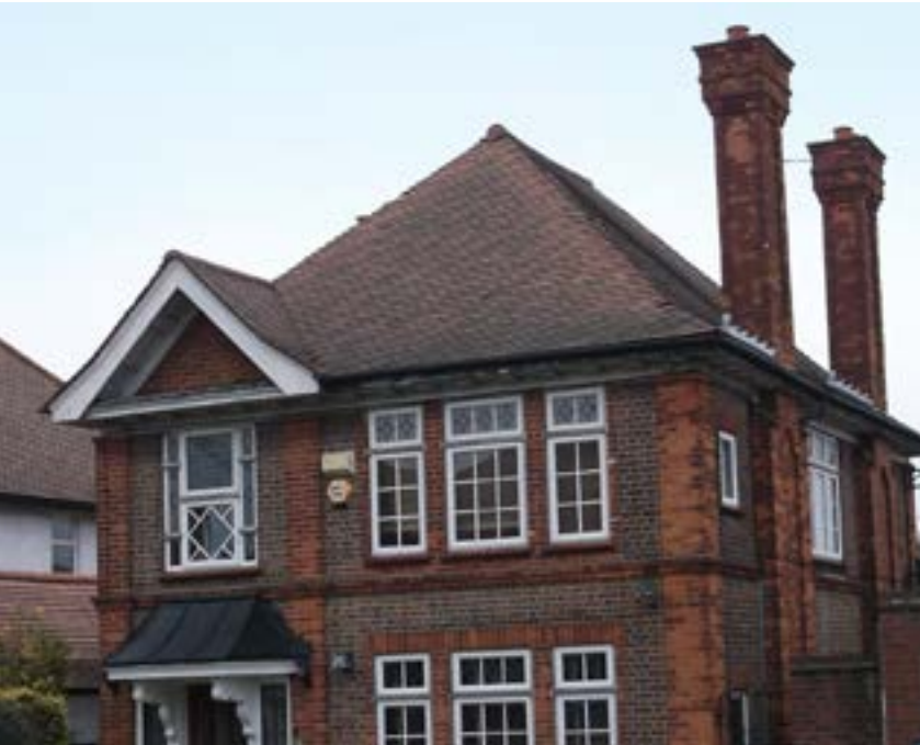
Figure 26: Decorative brick chimney at Sudbury Court
