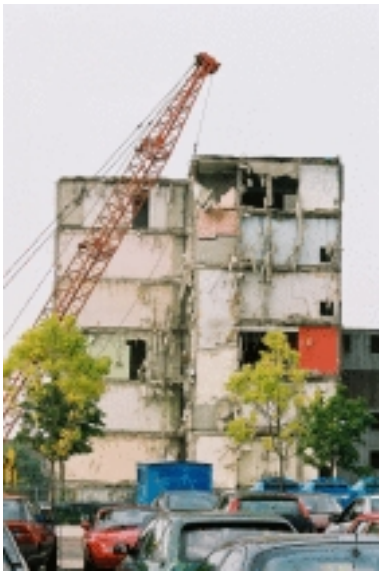
Demolition of building
