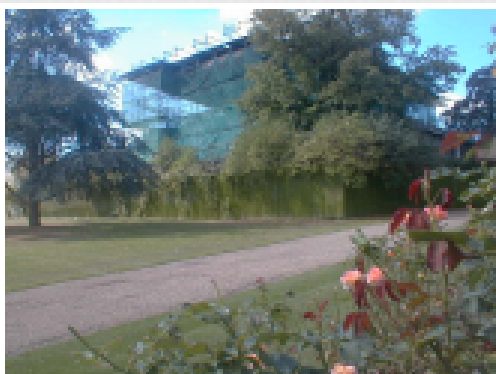
5. House viewed from the north east.
