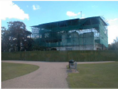
1. House viewed from the west.
