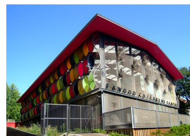
Picture 23 Fawood Children's Centre, Stonebridge.
