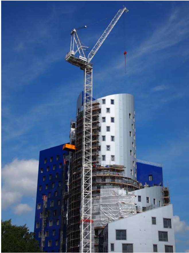
Picture 6.3 Student housing under construction in North End Road
