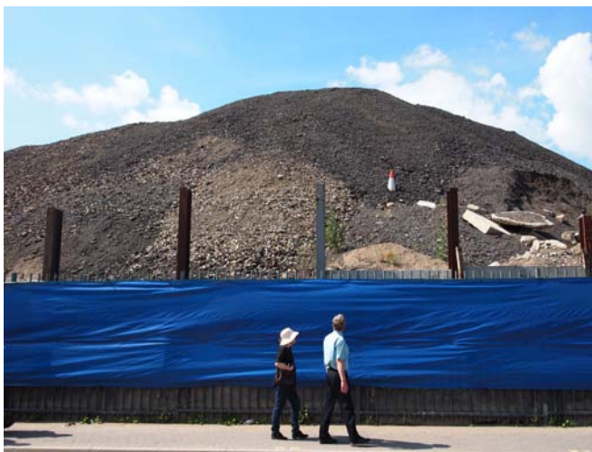
Picture 4.3 Waste storage on Hannah Close
