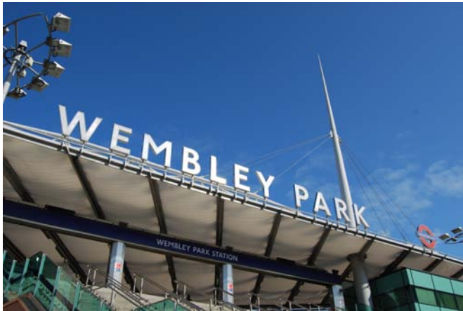
Picture 3.9 Wembley Park Station
