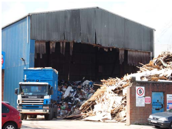
Picture 4.2 Waste management site, Fifth Way
