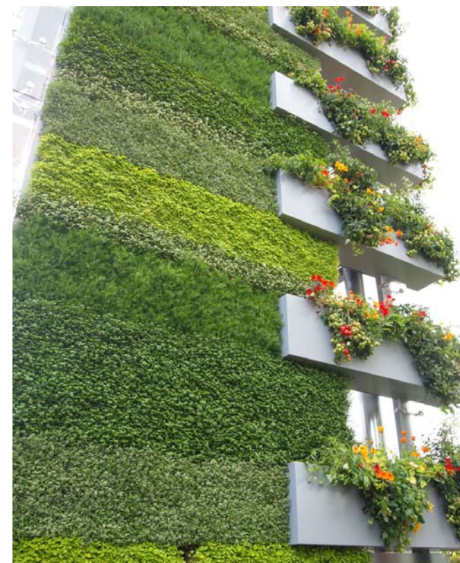
Picture 10.2 Living wall & planted balconies
