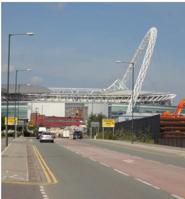
Picture 5.1 Stadium Access Corridor
