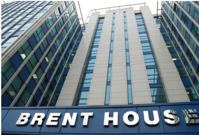
Picture 4.6 Brent House, Wembley High Road
