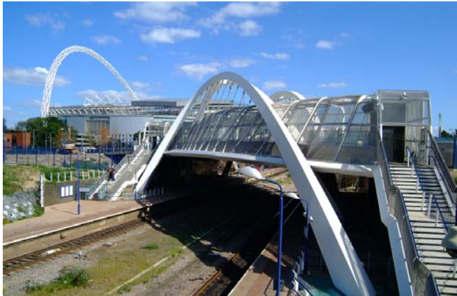
Picture 5.8 White Horse Bridge
