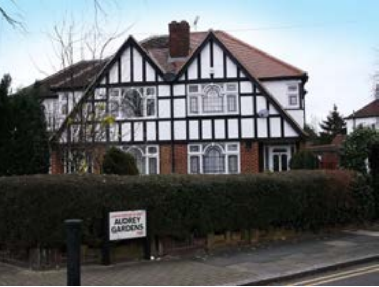
Figure 24: Half timbering at Sudbury Court
