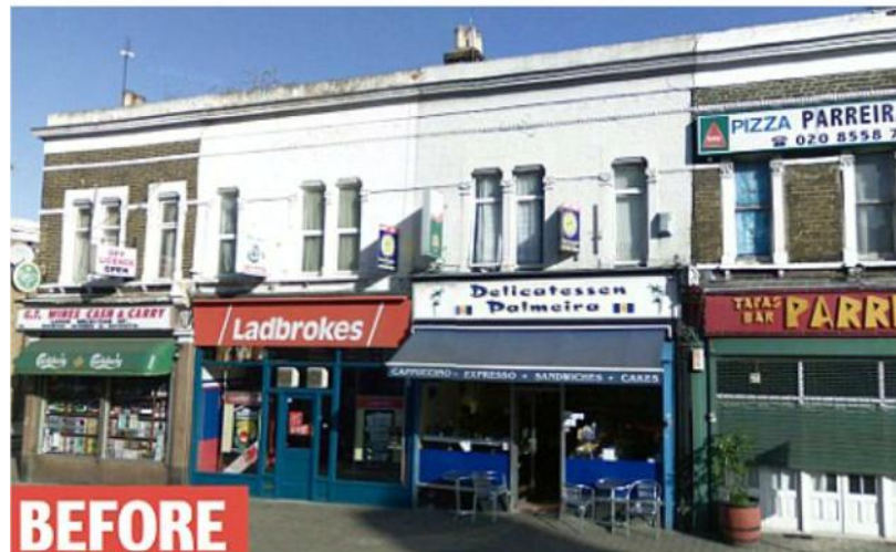
Figure 9: Example images of shopfront improvements along Leyton High Street
